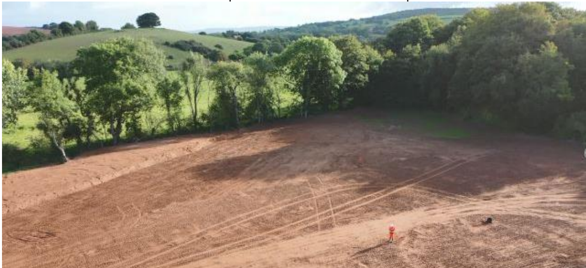
Drone Footage prior to final restoration [Vertase FLI]
