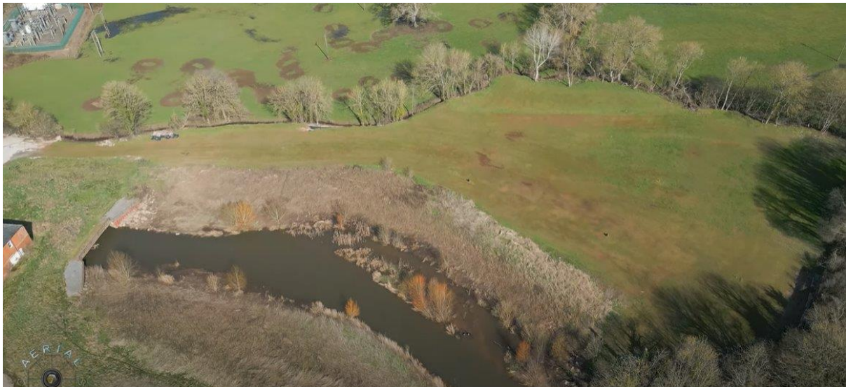
Aerial Drone Footage following restoration [Aerial Dimensions]
