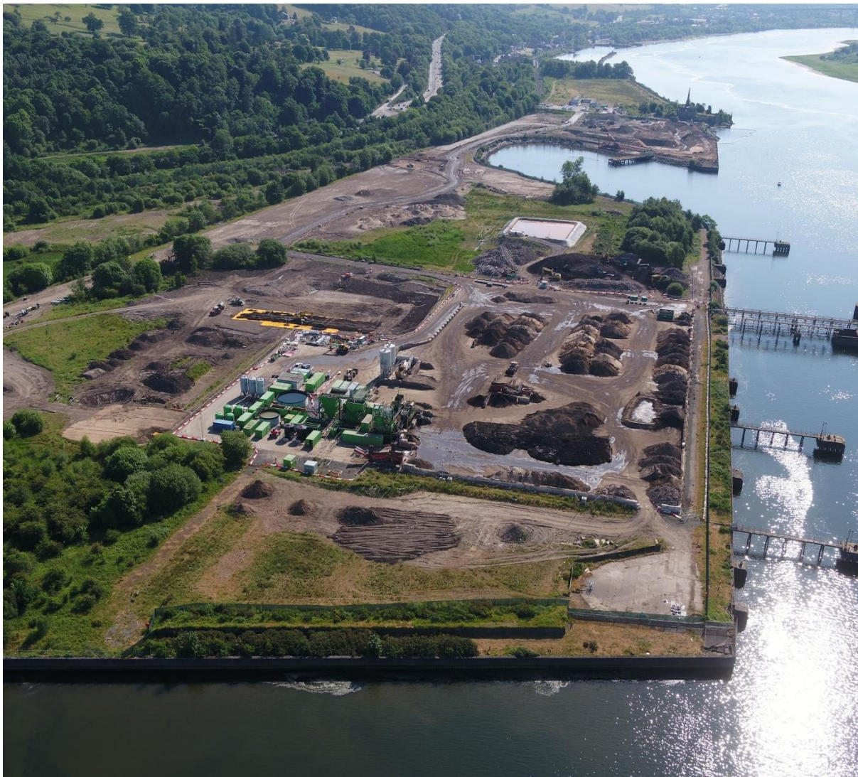
Aerial image of siteworks being undertaken. Credit: DEME.
