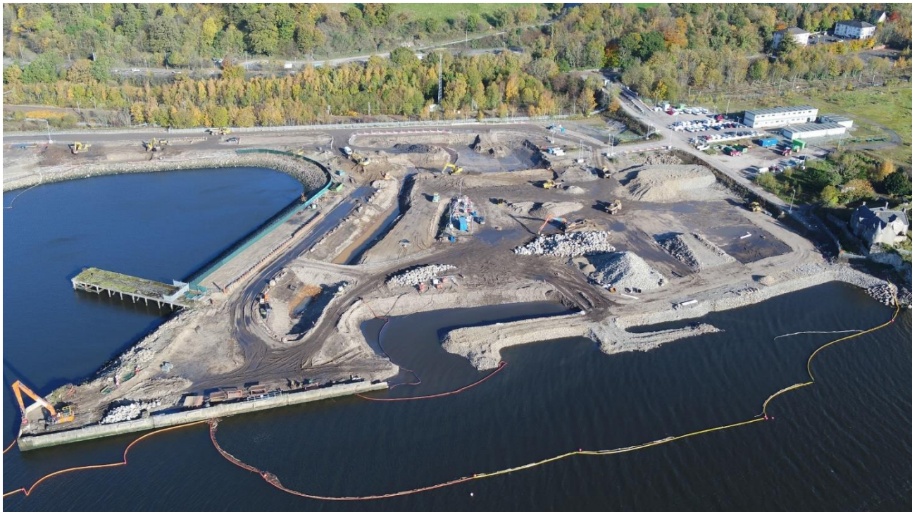
Aerial image of siteworks being undertaken. Credit: DEME.
