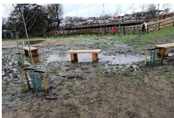
Poor soil management in the construction of an amenity area (Photo: ©Vaughan Redfern)
