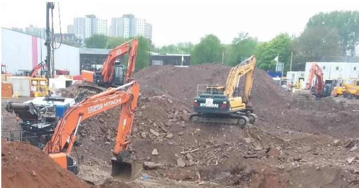
Remediation and soil recovery (Photo: ©Martin Ballard)
