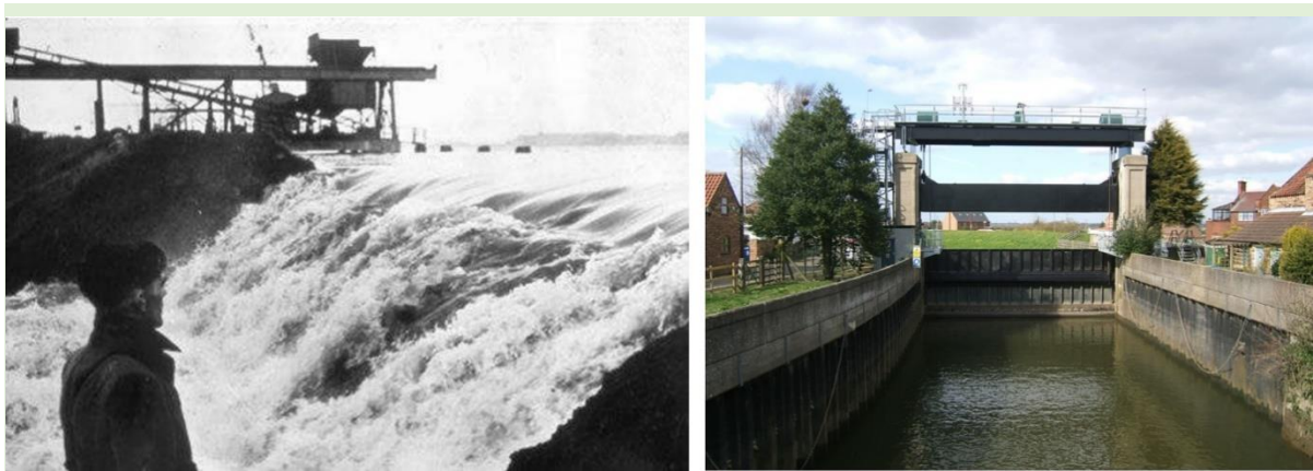
A breach at Erith after the North Sea flood (Photo: ©1953 UK Government (HMSO) 89 )
