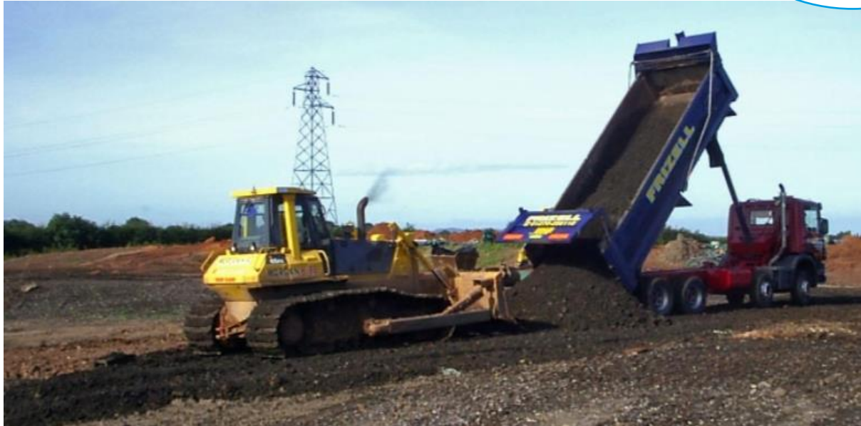
Disposal of hazardous ballast waste from rail network (Photo: ©Paul Dumble)
